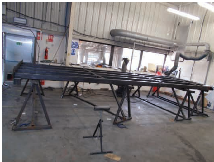
Secondary Steel Sub Frame Welding
